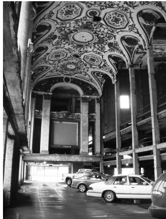
Michigan Theatre Parking Garage.
